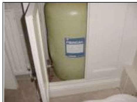
Factory lagged cylinder in bathroom on first floor
