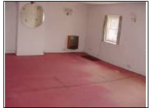
Dip in floor of top floor right room (all directions given as you face the front of the property)
