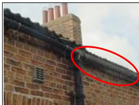
Asbestos guttering to rear
