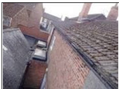
Doubling up of concrete tiles to rear
