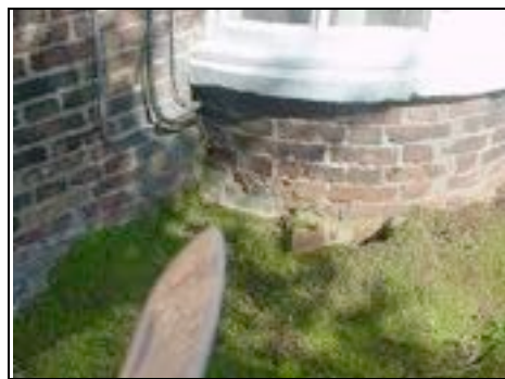
Cement repairs to base of semi-circular window
