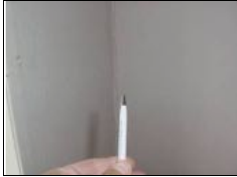
Top floor right bedroom. Crack between front wall and studwork.
