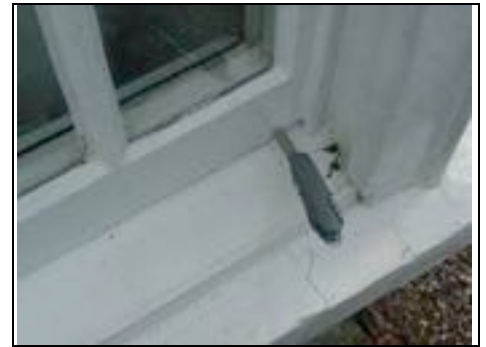
Wet rot in the front sliding sash window
