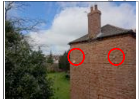
High level airbricks
