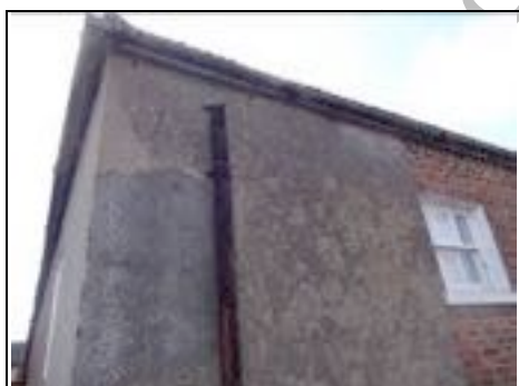
Believed to be disused soil and vent pipe to rear right corner
