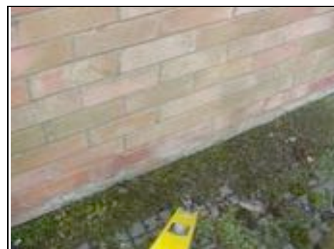
Stretcher bond brickwork
