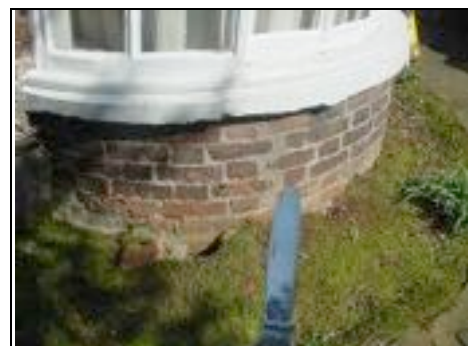
Crack to front bow window
