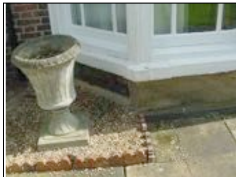
Deterioration to stonework under bay window
