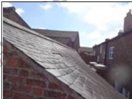
Twist in rear slate roof over garage
