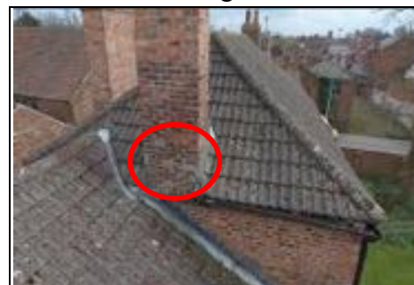
Poor quality cement repairs
