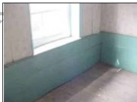
Top left room Floorboards running front to back therefore joists running side to side
