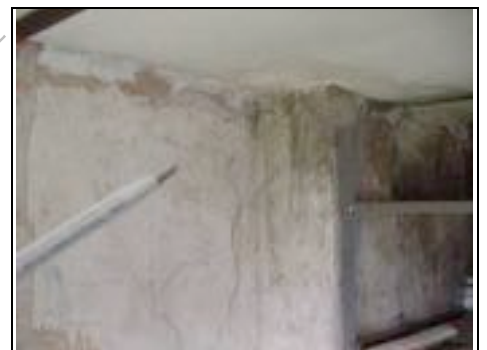
Chimney Two leaking top floor left bedroom
