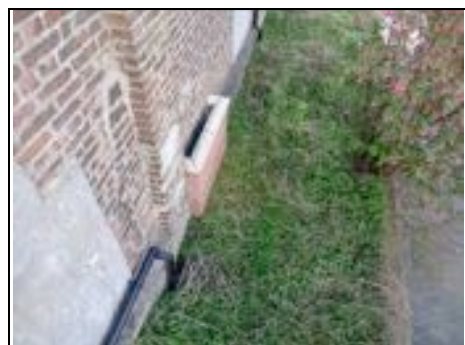
Window of cellar blocked to stop flooding
