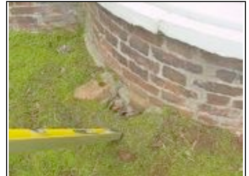
Airbrick to circular bay on right side
