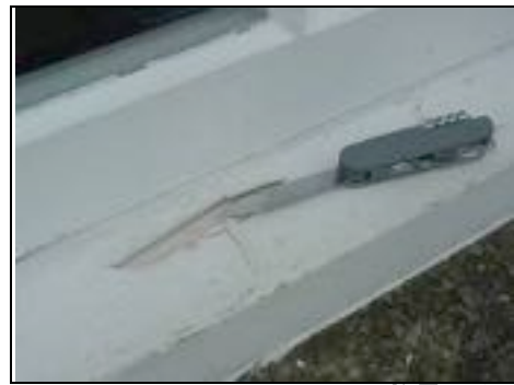
Cracking and there is general flaking of paintwork
