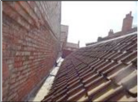
Valley gutter to rear of pantile roof
