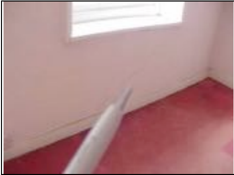
Top floor right room raking crack relating to movement to window below
