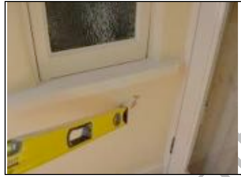
Modern plaster in conservatory not coping with seasonal movement in property
