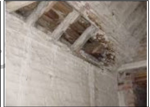
Valley gutter problems, part repaired in lead but needs double checking this is watertight
