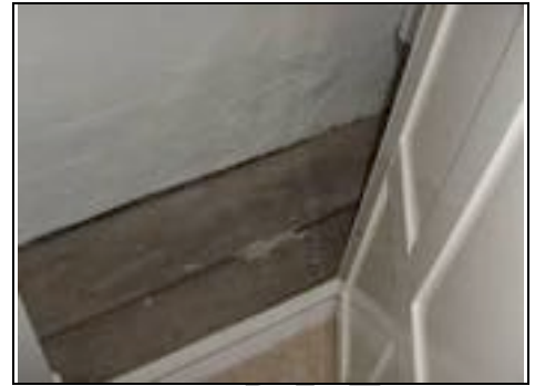
Floorboards in cupboards indicating joists run from front to back on first floor of left side of building
