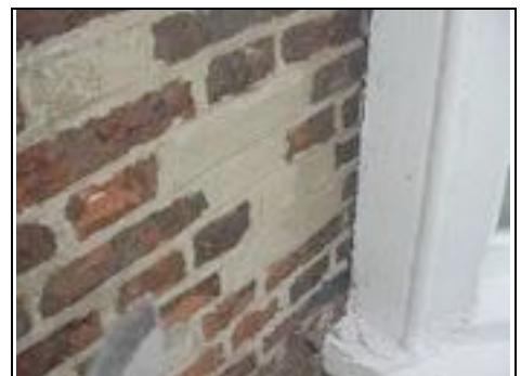
Cement repairs spotted dog effect to brickwork
