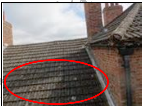
Spalling brickwork from chimney falling onto roof
