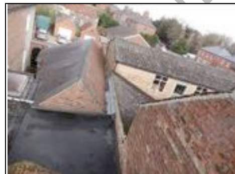
Slate roof, tiled roof and flat roof to rear
