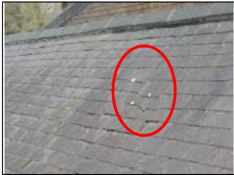
Tingles to slates on garage roof
