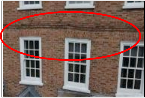
Movement/twist in brick string course and associated brickwork ~ Aerial View - 360 Photo ~
