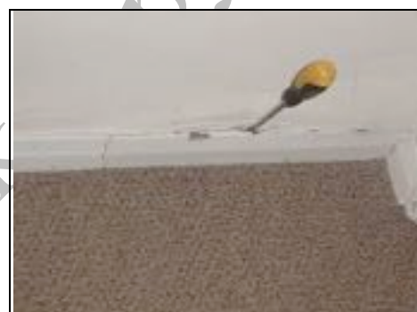
Possible wet rot or dry rot in utility room in left building
