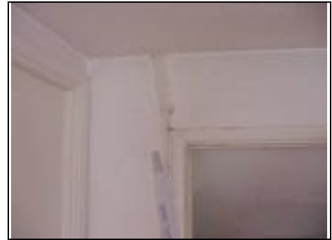
Top floor right bedroom cracking which we believe relates to movement to front wall and direction of joists discussed earlier
