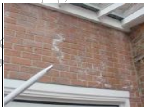
Efflorescence below parapet wall indicating it is allowing dampness in
