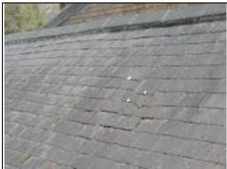
Tingles to slates on garage roof
