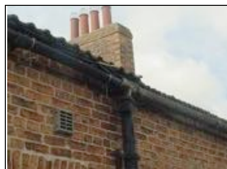
Asbestos guttering to rear
