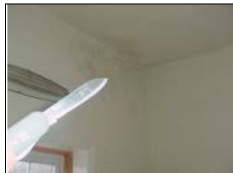
First floor far left bedroom dampness coming in underneath concrete tiled roof with tiles that are wrongly gauged.
