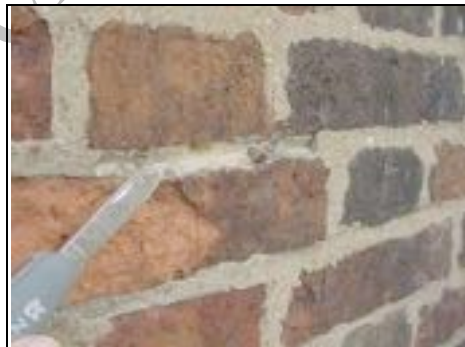
Cement mortar with lime underneath causing spalling to brickwork
