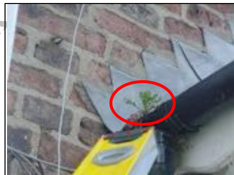
Vegetation growing out of gutters and general lack of maintenance
