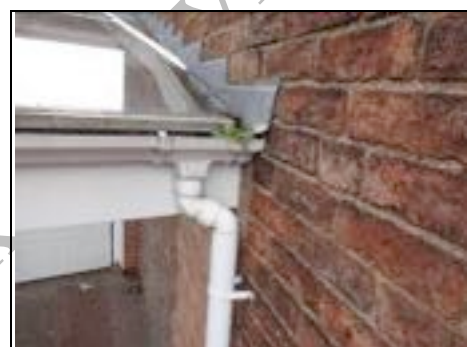
Plants growing out of guttering
