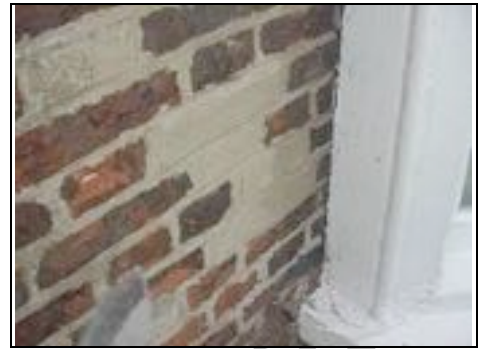
Cement repairs
