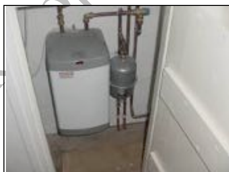
Water softener on first floor of left building
