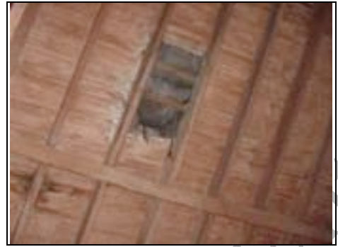
Damage to garage/workshop roof
