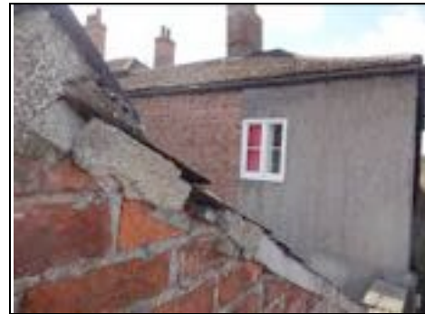
Verge needs repointing to the slates of the garage roof
