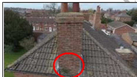
Right chimney Poor quality repairs and plant growing
