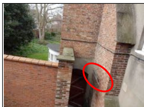
Bonding timber to right side of property
