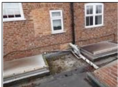
Soil and vent pipe to rear of property
