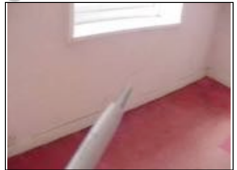
Cracking below window in right room
