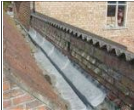
Valley gutter repaired that was allowing dampness into garage
