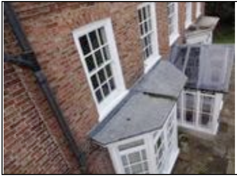
Front left lead bay window roof
