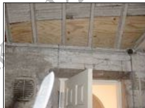
Timber lintel in coal bunker which indicates there may be other timber lintels
