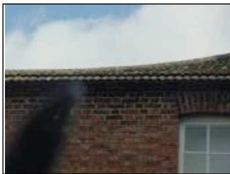
Badly gauged/tipping of concrete tiles/no tilting fillet to left side of front roof
