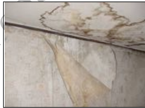
Leak to top floor left bedroom
