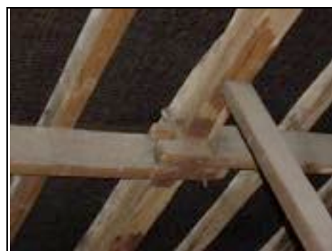
Strengthening 'braces' on purlins
