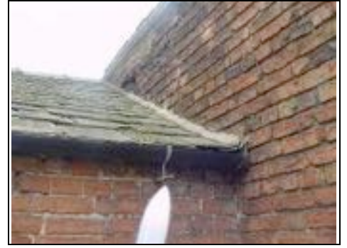
Cement mortar to flashing of stables
