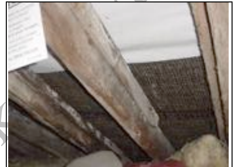
Breathable protective underlayer indicating modern alterations as well as hessian felt
